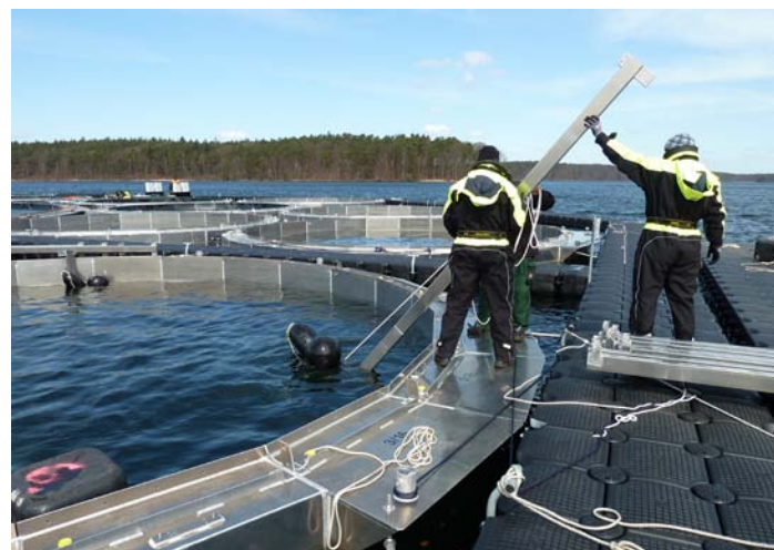
Fig. 2: The LakeLab under construction in early spring 2012. ©IGB
